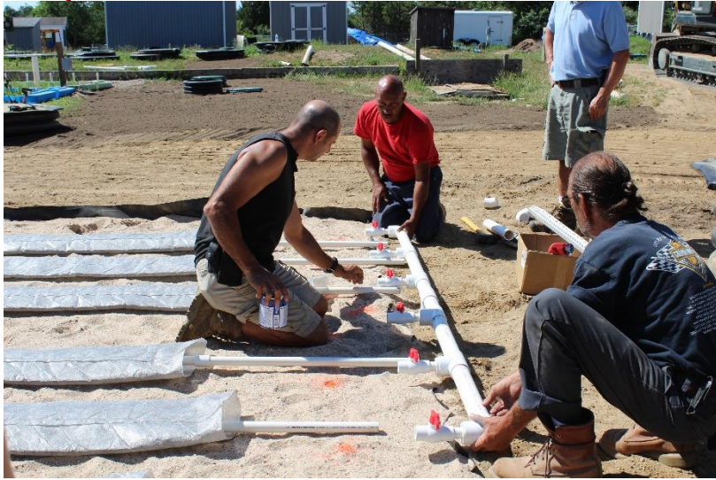
Manifold installation
