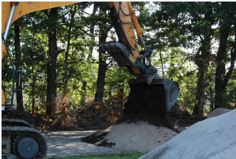
denitrification layer mixing FAR BEYOND 50/50 sand/woodchip
